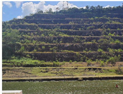
Terraced hillside to prevent erosion
