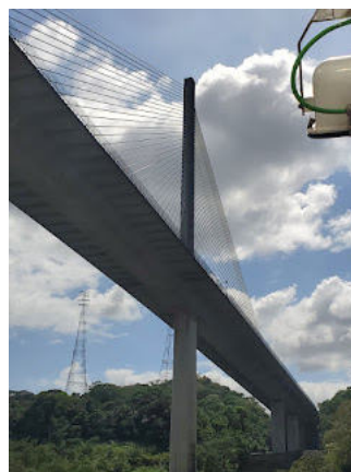
Centennial Bridge, close to area of the Continental Divide
