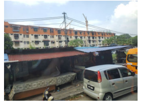
Typical apartment housing
